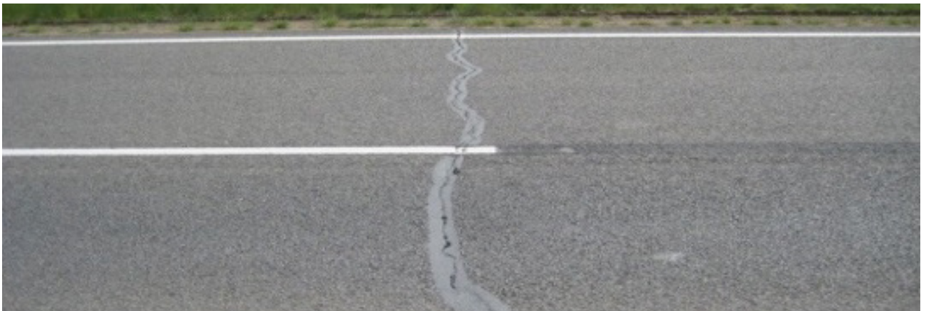
Longitudinal and transverse cracking
