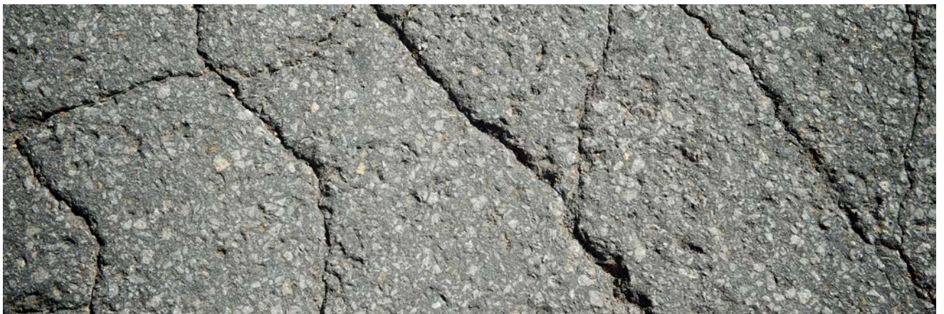
Alligator cracking
